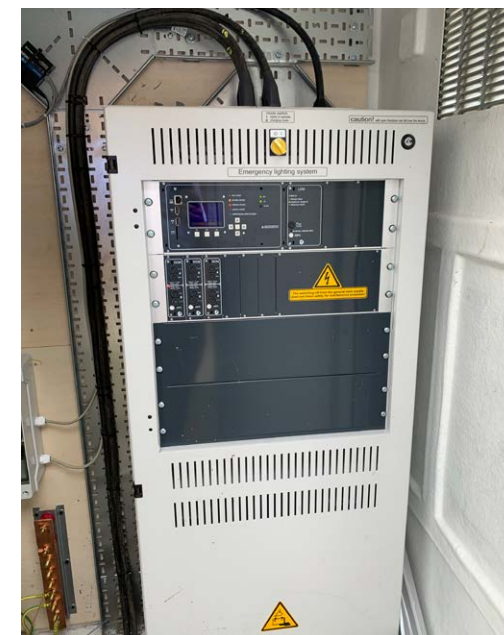
Figure 30. Installing an external battery system for emergency lighting means that the emergency lighting system can be built into the sports lighting system without needing to demount the netting system to test and replace emergency lighting batteries.
