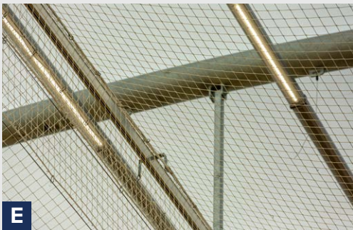
Figure 21. Design elements of the tensioned net cage at the Bradford Park Avenue facility: A - the bottom of the net is laced to a tensioned steel wire rope secured to a concrete ring beam in the floor; B - the corners of the tensioned net area are wrapped externally to protect the net and fixings, and internally (not shown) to prevent balls being trapped in the corner during matchplay; C - an external view showing the overlap of the superstructure outside the tensioned net area; D - the corners of the net are attached to the superstructure using tensioned chains and cables; E & F - the horizontal roof net arrangement around the trackway for the pull out practice nets and below the sports lighting system; G - corner protection in place for player safety and to stop balls getting trapped.
