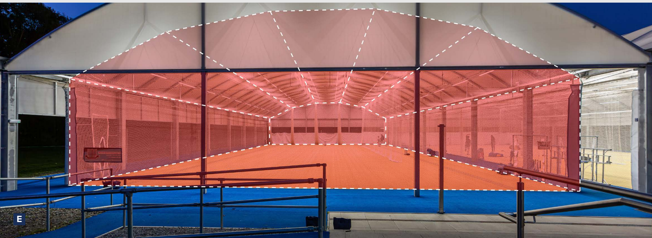
Figure 20. By fixing the roof of the tensioned net area over and around the trackway for the practice nets, the roof line of the tensioned net area can follow the roof line of the superstructure. This can create a better match play experience for users by increasing the volume for lofted straight shots with the bat.
